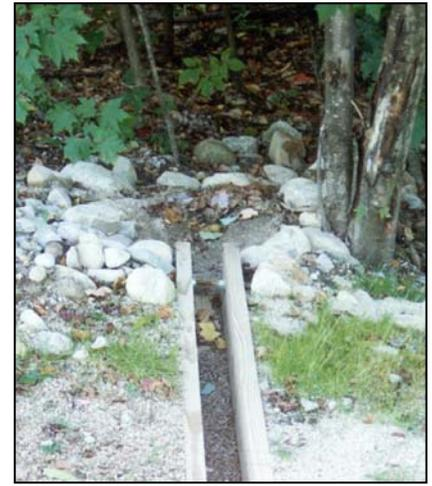
Install the culvert flush with the surface of the road. If placed too high, stormwater will not enter the structure; if placed too low, it may quickly fill with road material and sediment loosened during installation.
