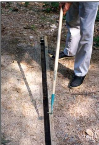
**Maintenance:** Open-top culverts need to be cleaned regularly to remove sediments, gravel, leaves, and twigs. Check after storm events for accumulated sediment. A child's toy hoe fits easily into the culvert and can be used for cleaning.
